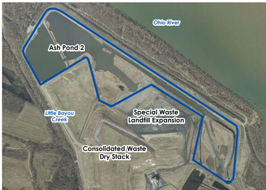
Figure 1 Ash Pond 2 Boundary
