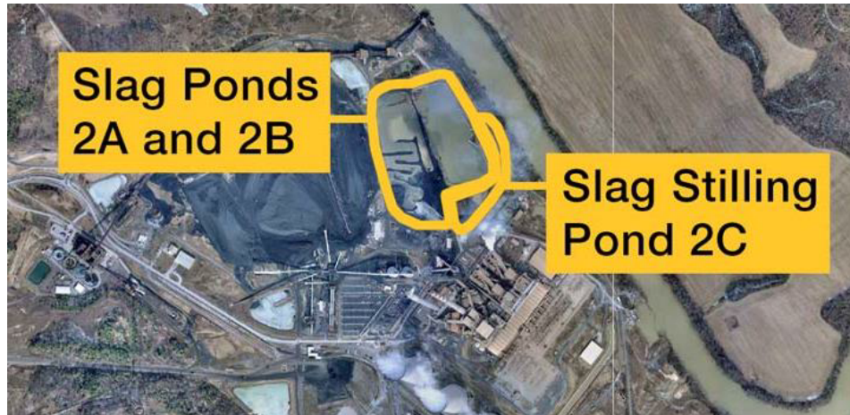
Figure 2. Aerial View of Slag Pond Complex
