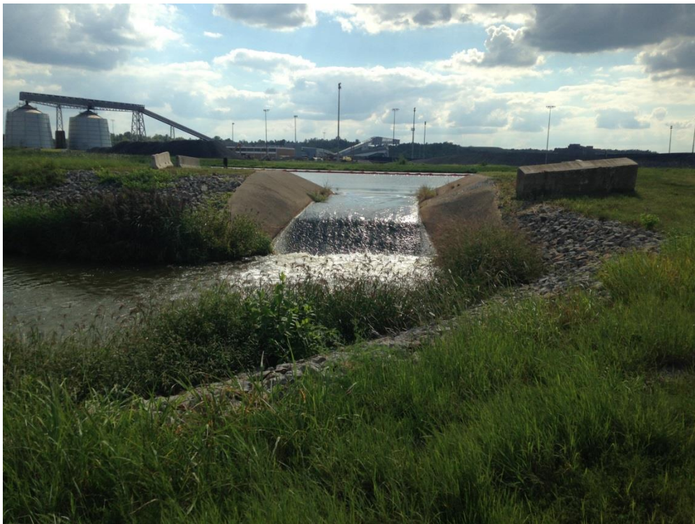
Photo 8 – Slag Stilling Pond 2C flume spillway outlet
