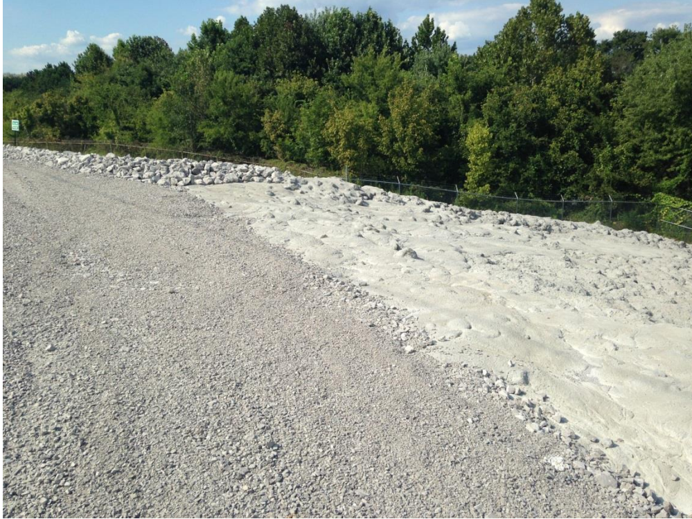
Photo 9 – Slag Stilling Pond 2C Emergency Spillway
