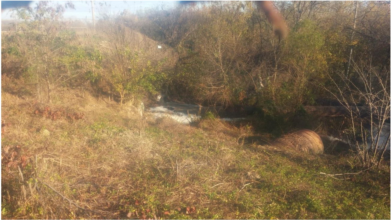
Photo 15 – Slag Stilling Pond 2C spillway outlets
