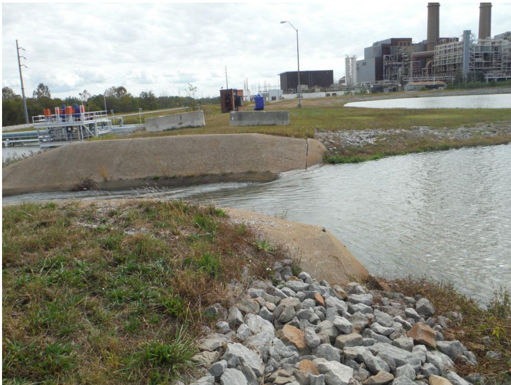
Photo 6 – Slag Pond 2B flume spillway inlet
