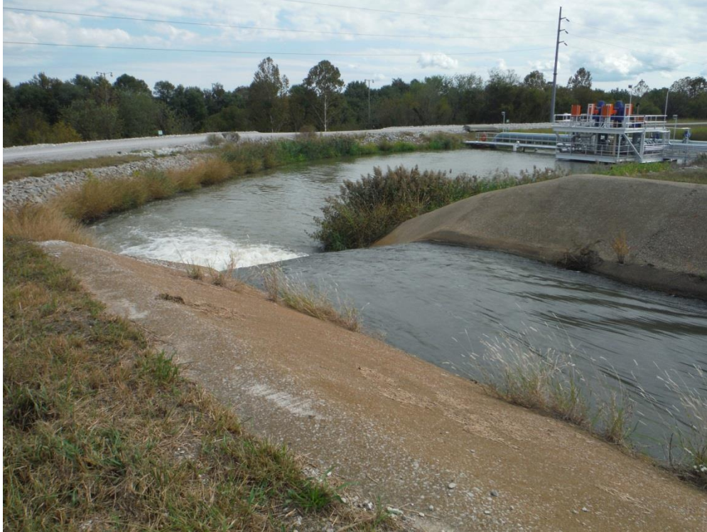
Photo 7 – Slag Pond 2B and Slag Stilling Pond 2C flume spillway
