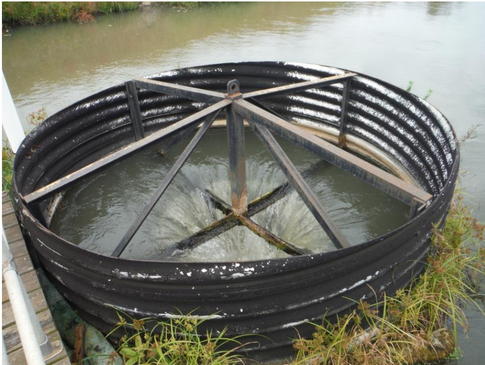
Photo 12 – Slag Stilling Pond 2C spillway skimmer, north
