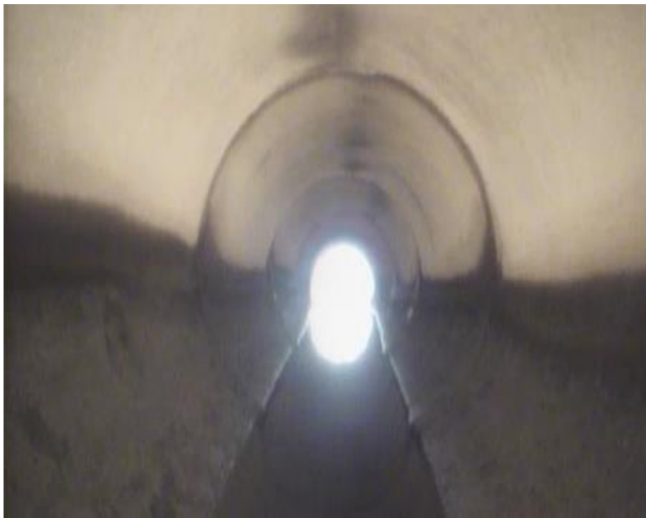
Photo 16 – Flow inside 36" concrete pipe (Typ.)
