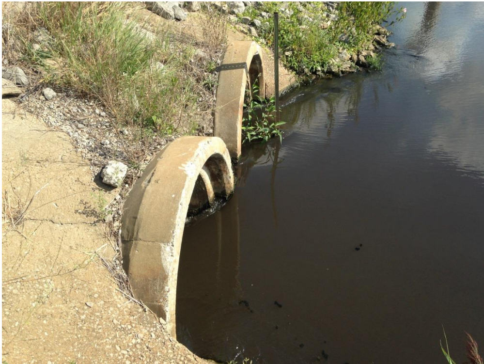
Photo 4 – Slag Pond 2A 48” spillway inlets
