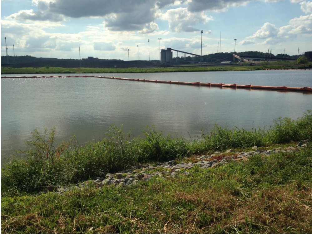
Photo 5 –Slag Pond 2B dike east dike condition
