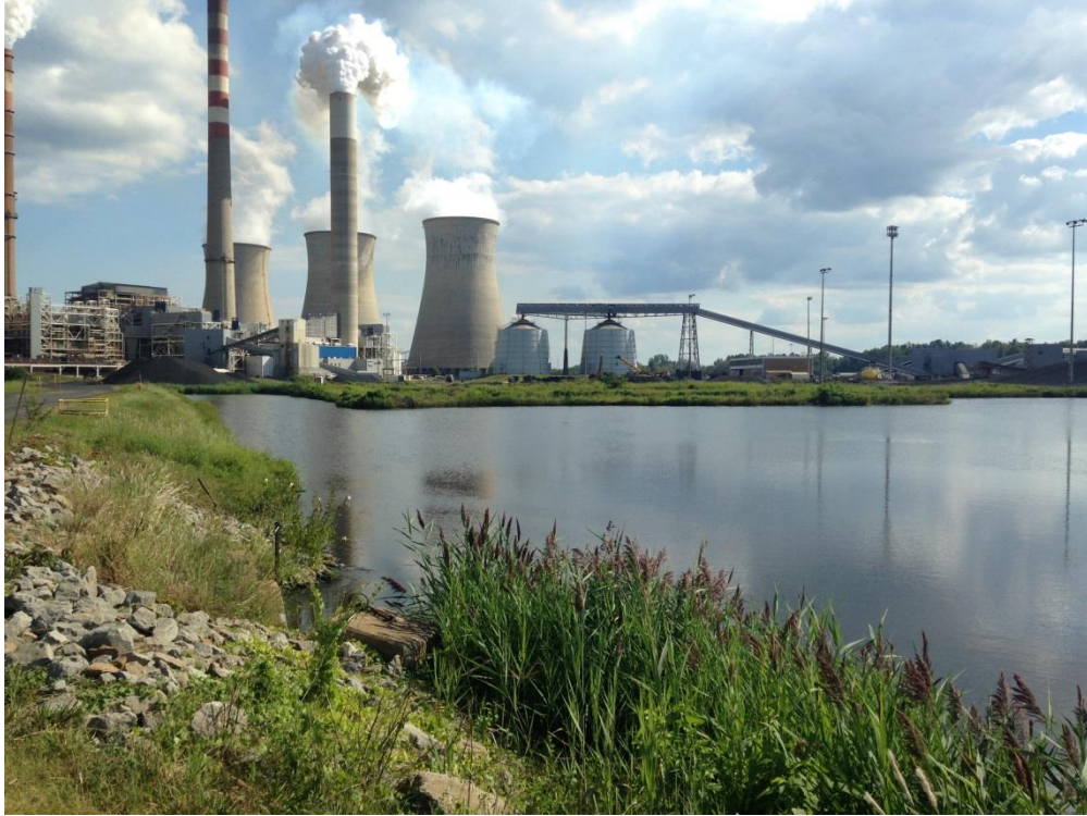
Photo 1 – Slag Pond 2A & 2B splitter dike condition, west side
