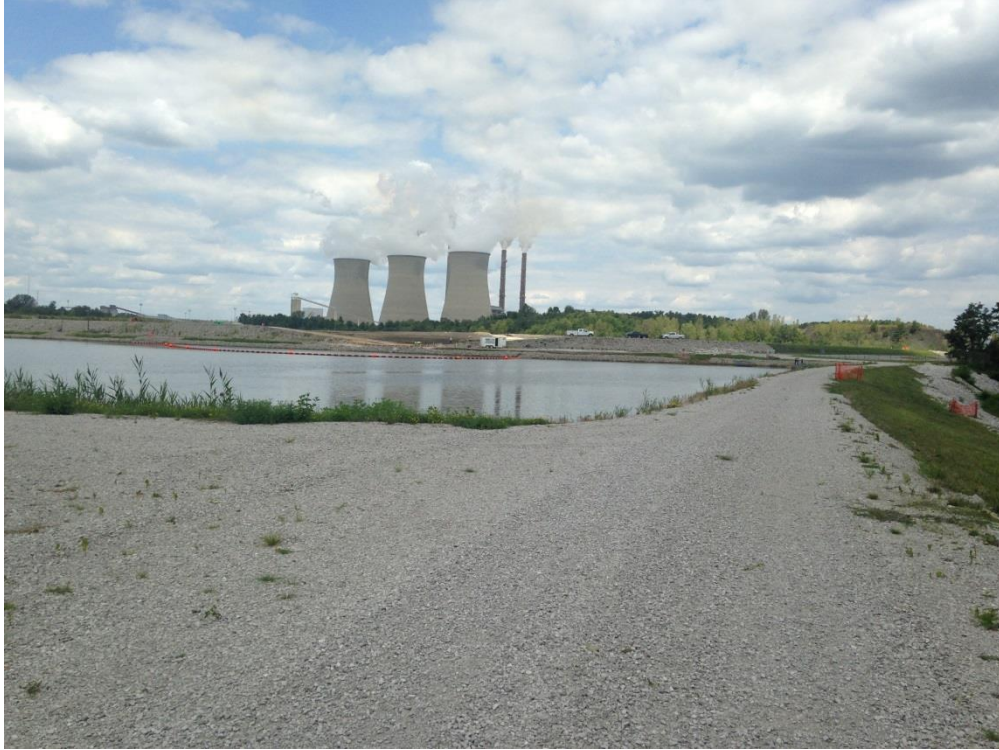
Photo 5 – East dike condition
