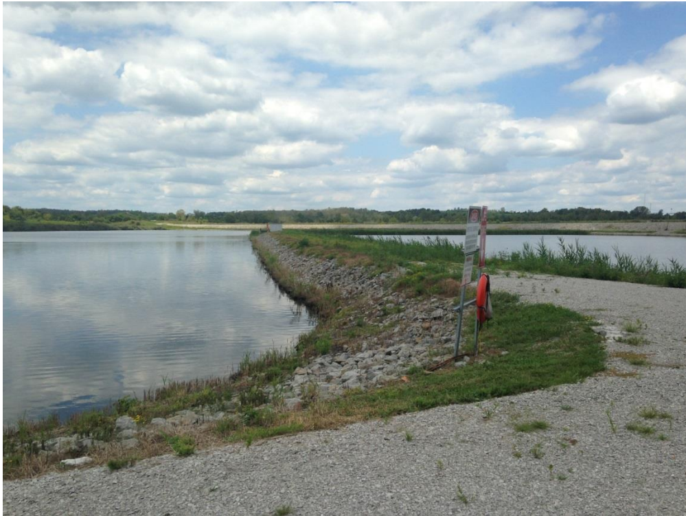
Photo 4 – Stilling Pond dike condition
