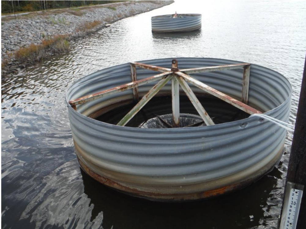
Photo 11 – Spillway skimmer, middle and south
