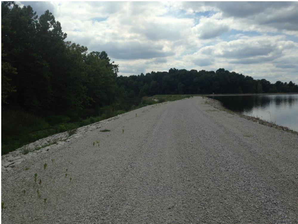
Photo 2 – Southeast dike condition
