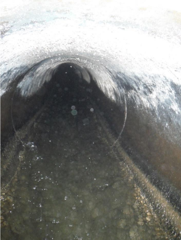
Photo 16 – Flow inside 36” concrete pipe (Typ.)
