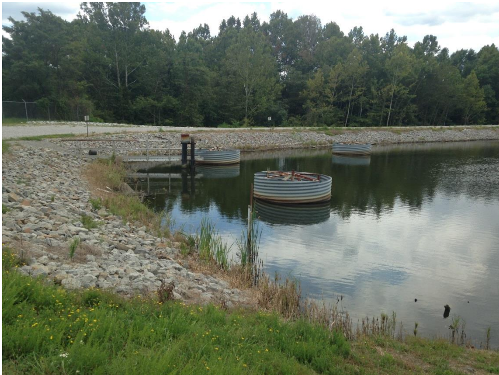
Photo 6 – Northeast dike condition
