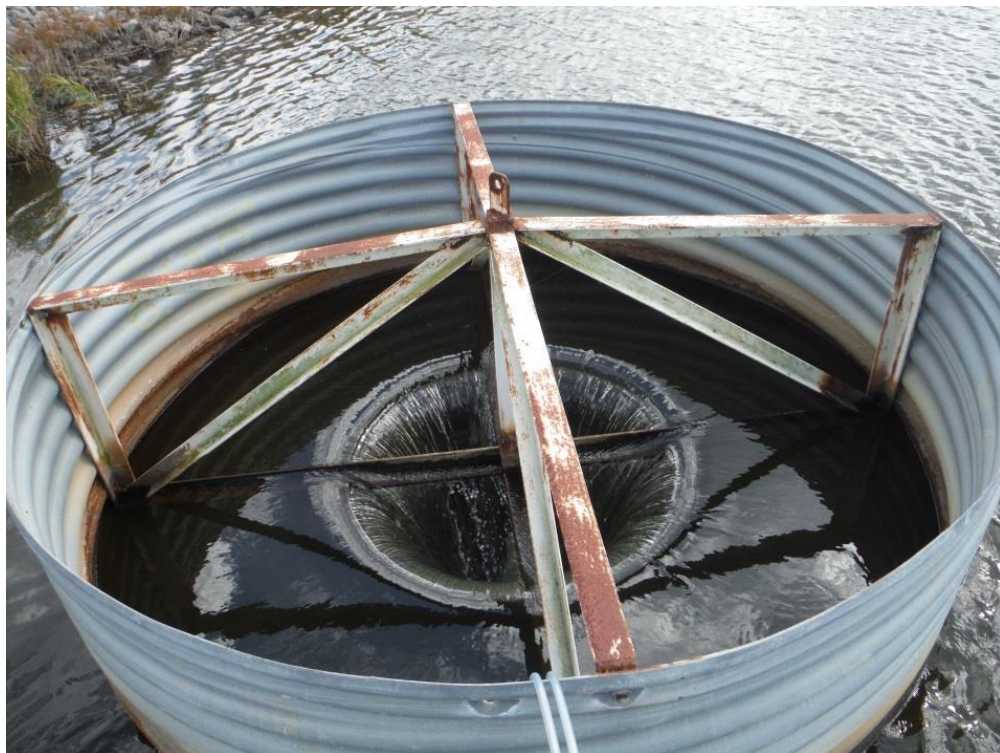
Photo 12 – Spillway skimmer, middle (Typ.)
