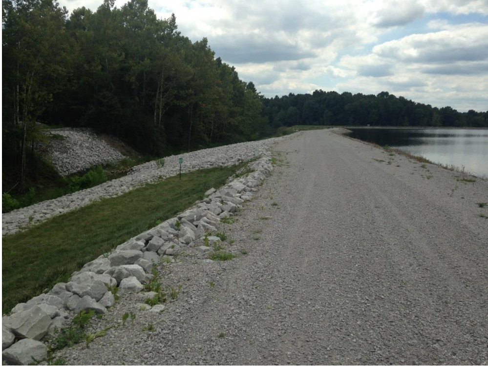
Photo 3 – East dike condition
