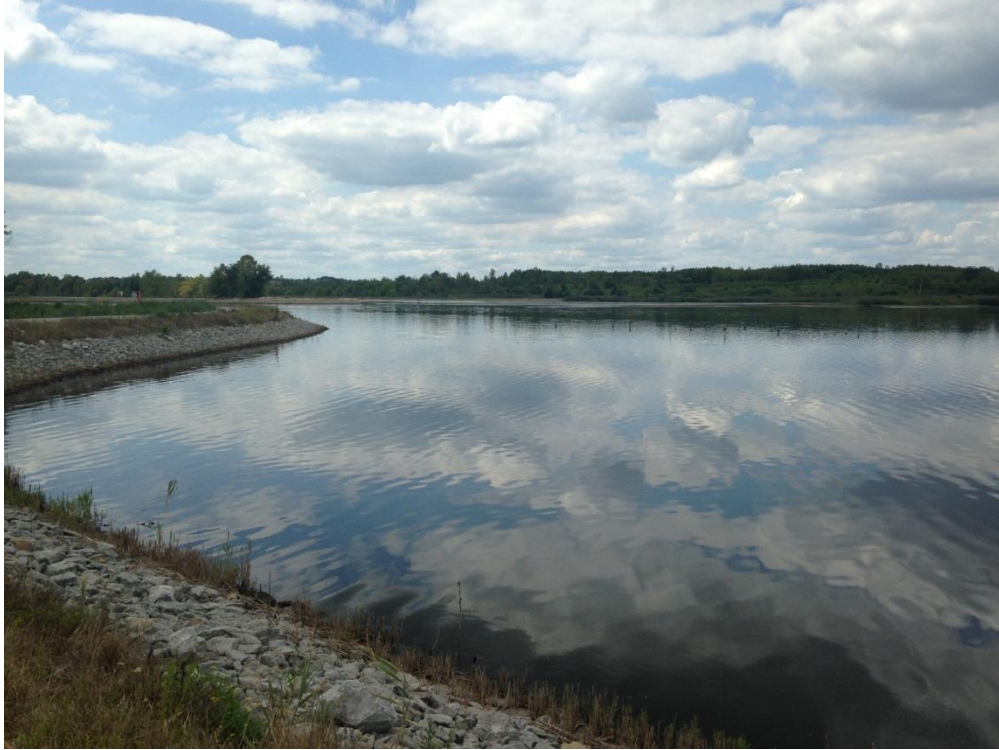
Photo 1 – Southeast dike condition
