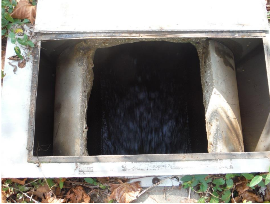
Photo 15 – Access location near outlet end of 36” concrete pipes (Typ.)
