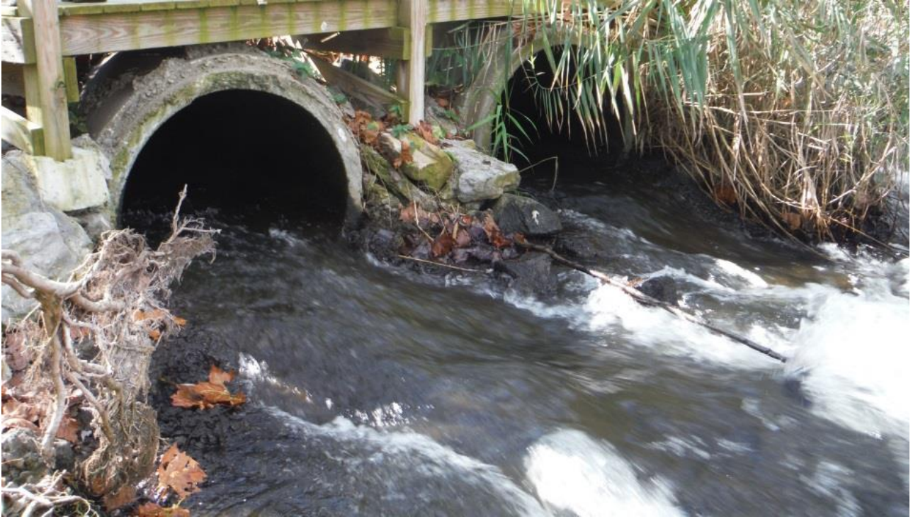
Photo 13 – 36” Pipe spillway outlets (east)
