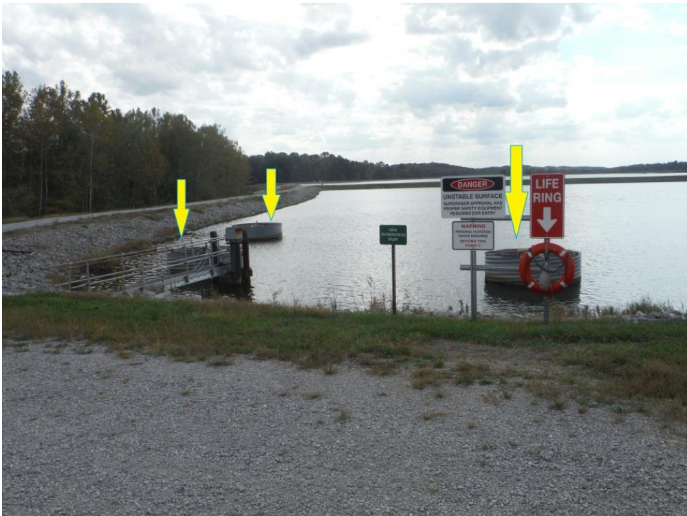
Photo 10 – General view of risers
