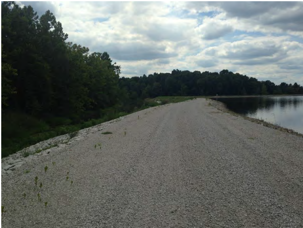
Photo 2 – Southeast dike condition
