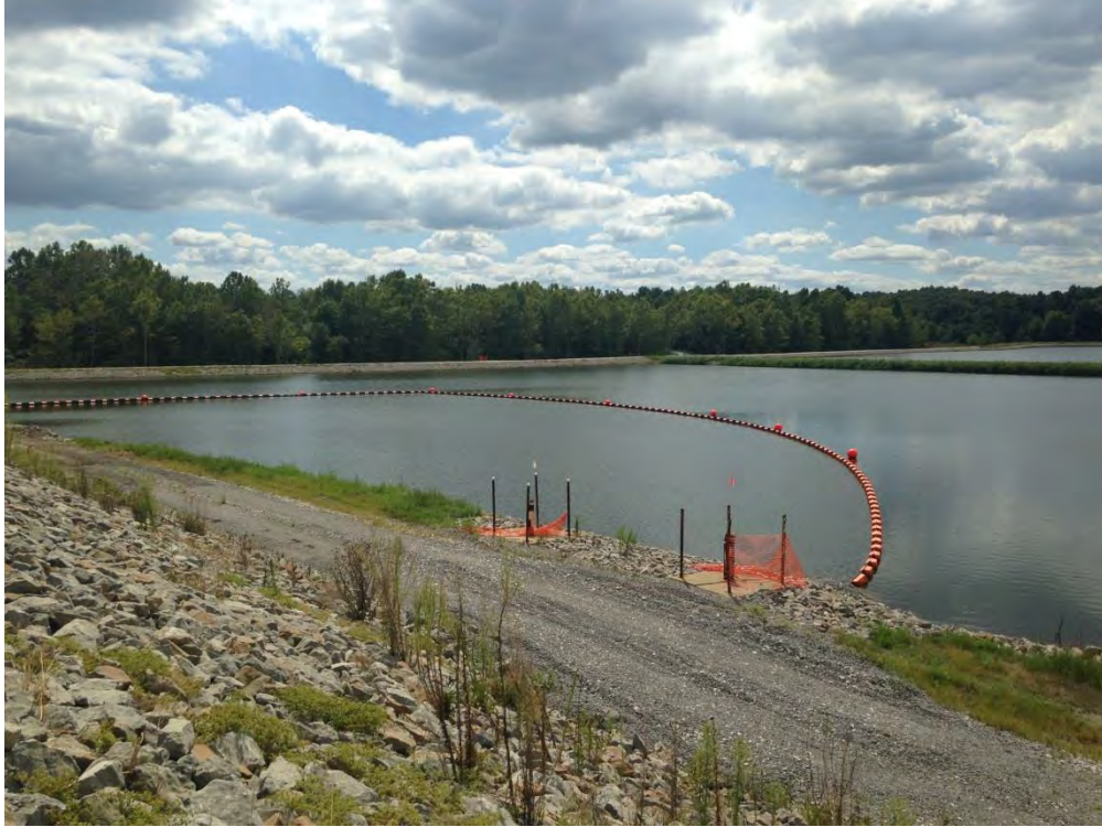
Photo 7 – North dike condition
