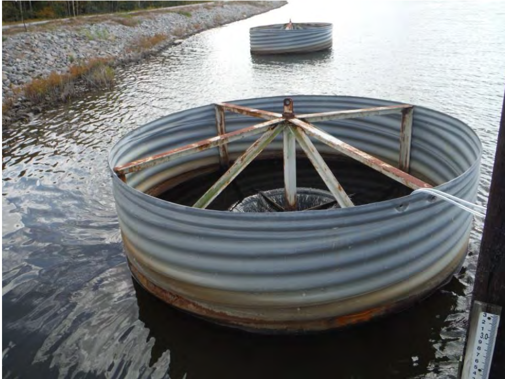
Photo 11 – Spillway skimmer, middle and south
