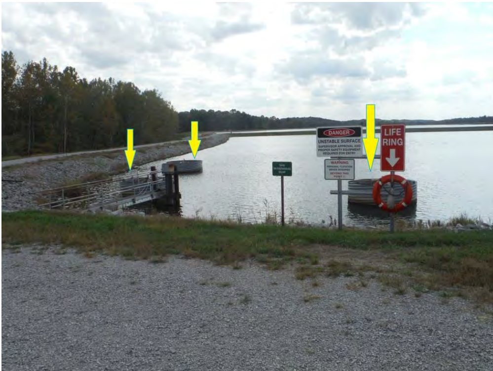
Photo 10 – General view of risers
