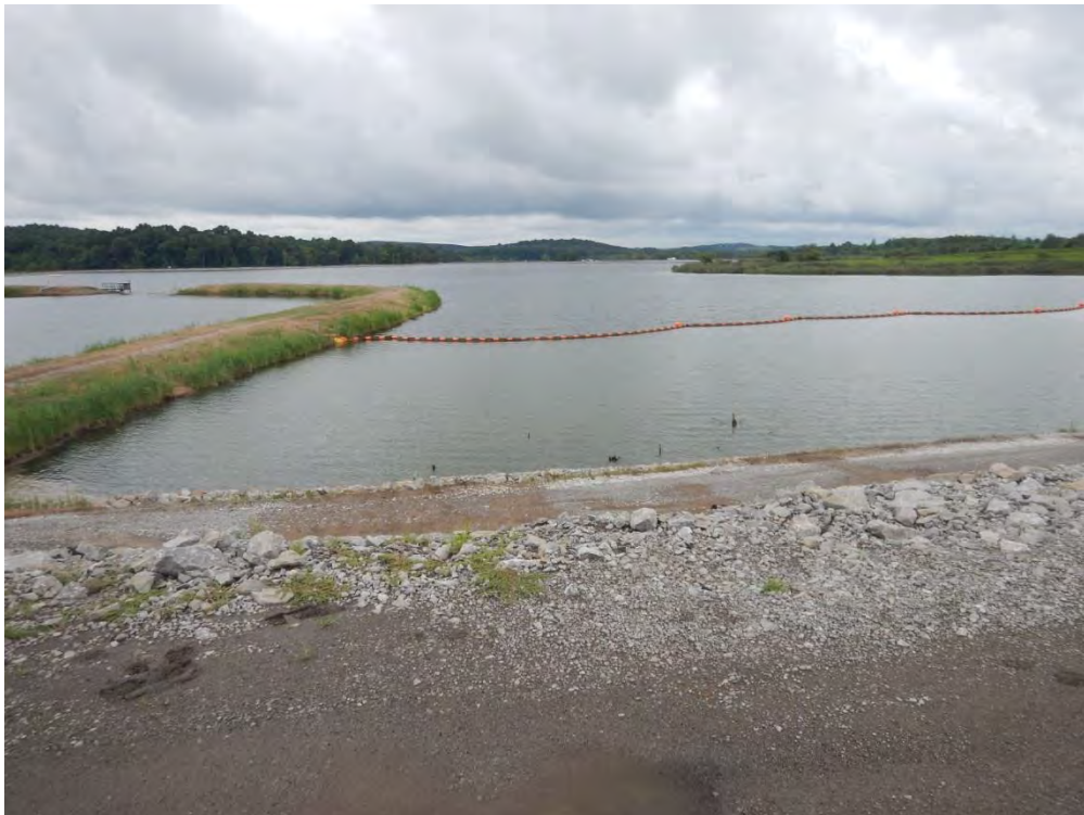
Photo 8 – North dike condition
