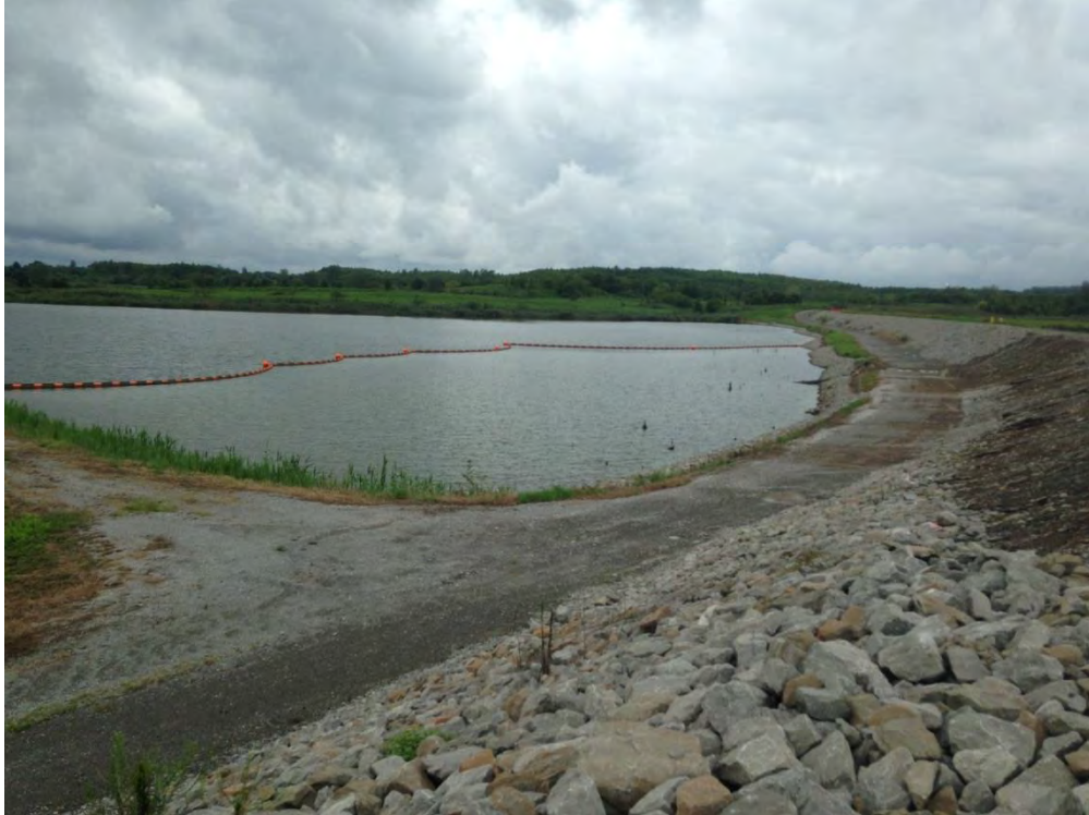
Photo 9 – North dike condition
