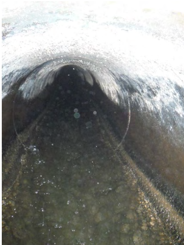
Photo 16 – Flow inside 36” concrete pipe (Typ.)
