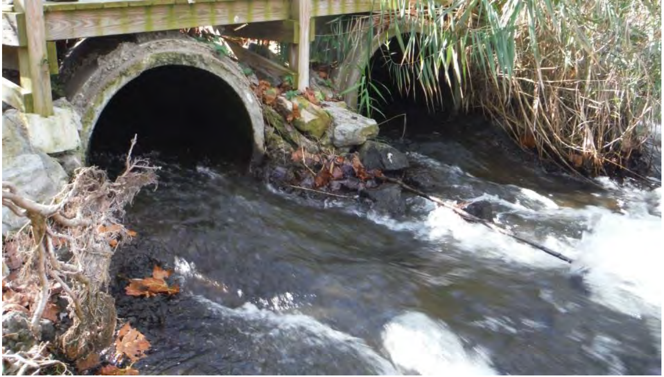
Photo 13 – 36” Pipe spillway outlets (east)
