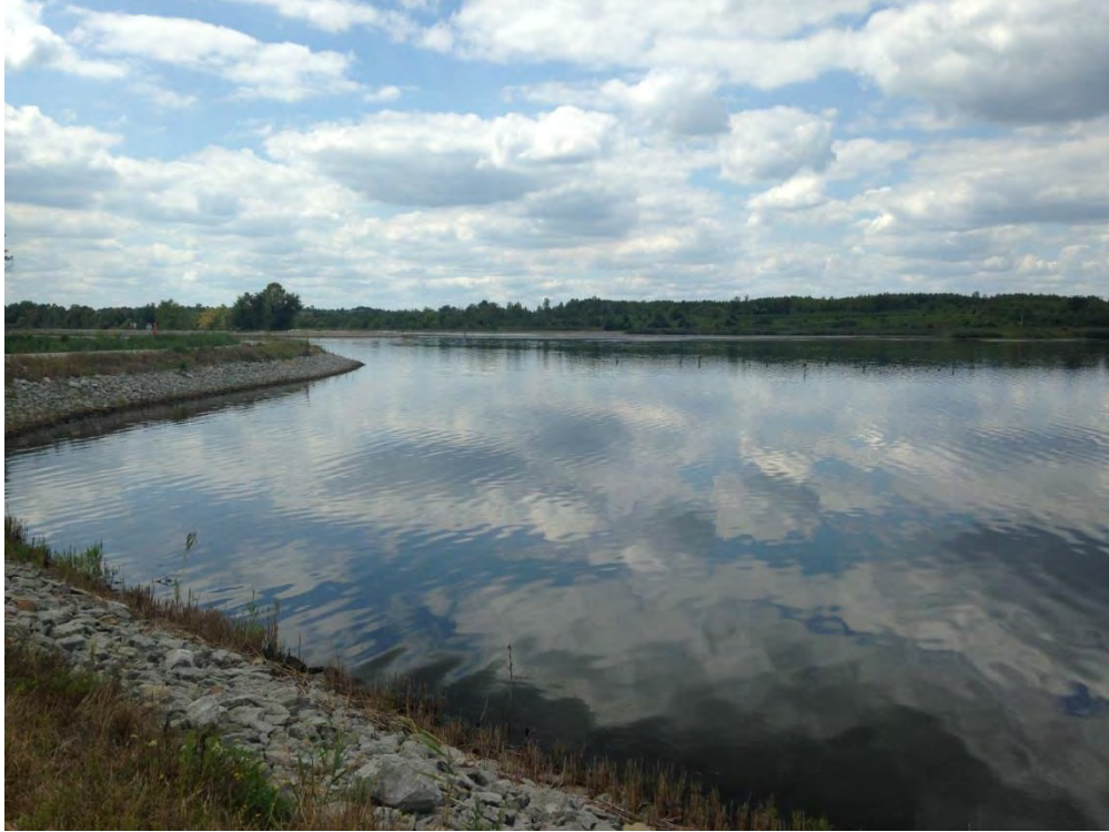
Photo 1 – Southeast dike condition
