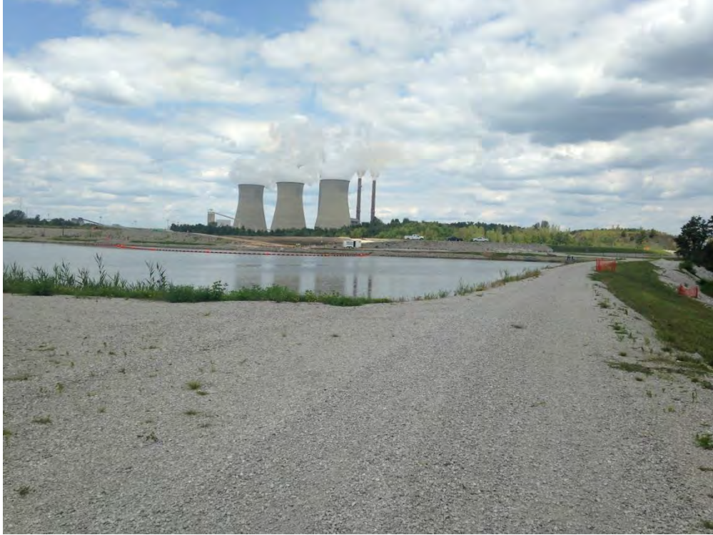
Photo 5 – East dike condition
