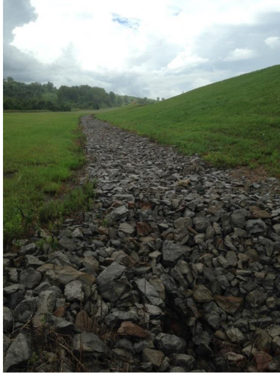
Photo 1 –Gypsum Disposal Area southern dike, looking west
