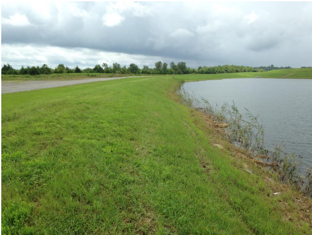
Photo 6 – Stilling Pond 2 south dike, looking southwest
