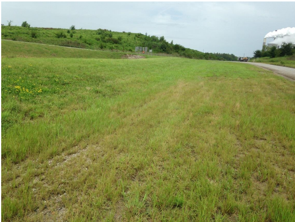
Photo 8 – Stilling Pond 2 south dike, looking northeast
