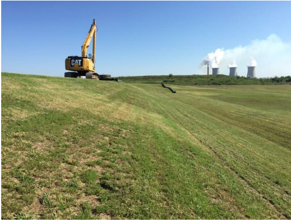
Photo 5 – Divider dike between Stilling Pond 1 and 2, looking east
