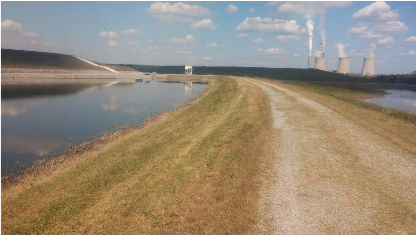
Photo 3 – Divider dike between Stilling Pond 1 and 2, looking northeast
