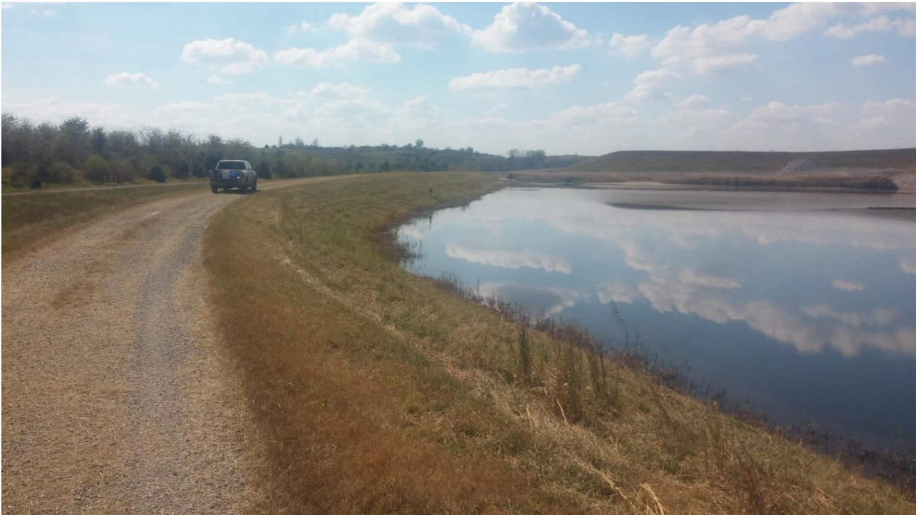
Photo 2 – Divider dike between Stilling Pond 1 and 2, looking southwest
