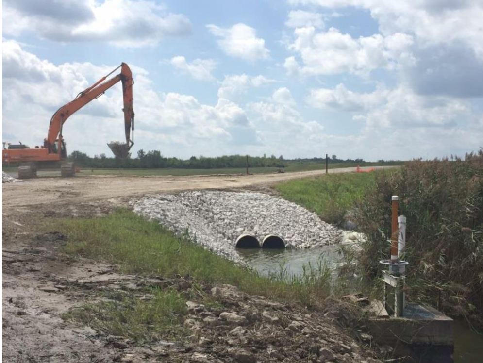
Photo 9 – Stilling Pond 2 Outlet, two 42” steel culverts
