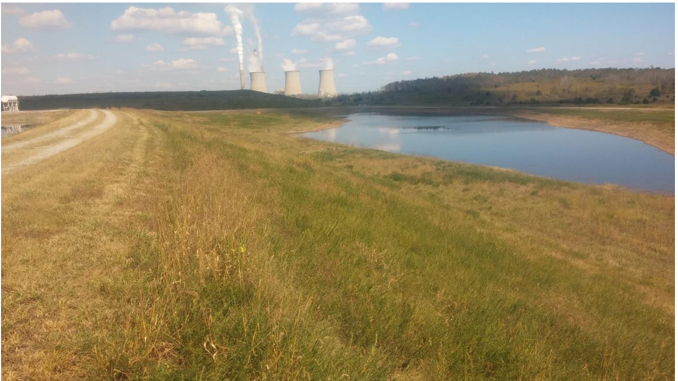
Photo 4 – Divider dike between Stilling Pond 1 and 2, looking east
