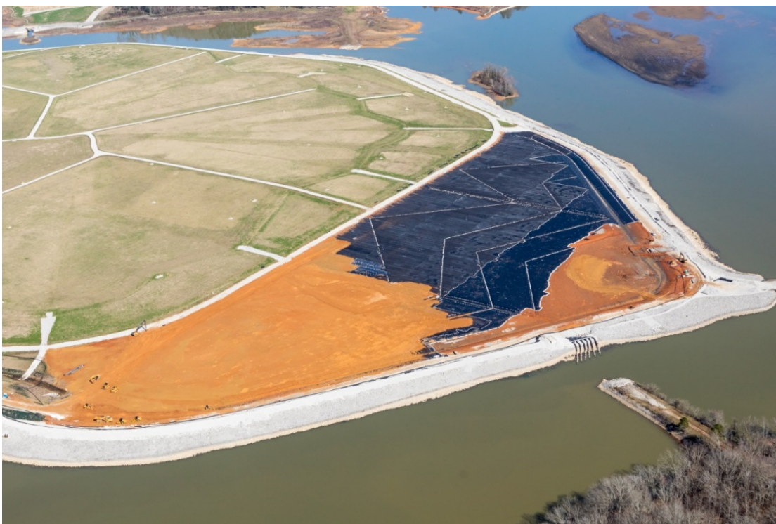
Figure 1 Aerial Photograph of KIF Stilling Pond Closure (February 27, 2018)
