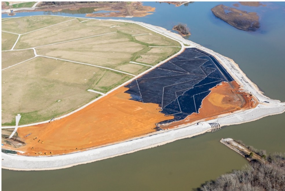
Figure 2 Stilling Pond Closure Construction (February 27, 2018)
