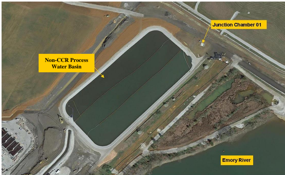
Figure 2: Current Site Conditions
