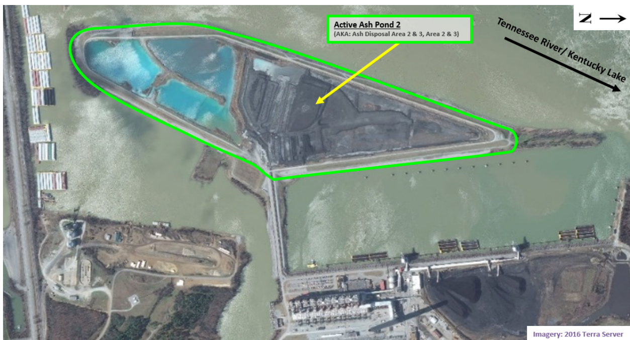
Figure 1 Active Ash Pond 2 Approximate Boundary
