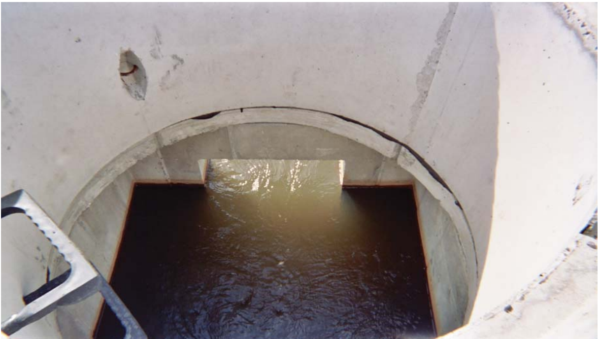
Picture 8: New drainage structures
