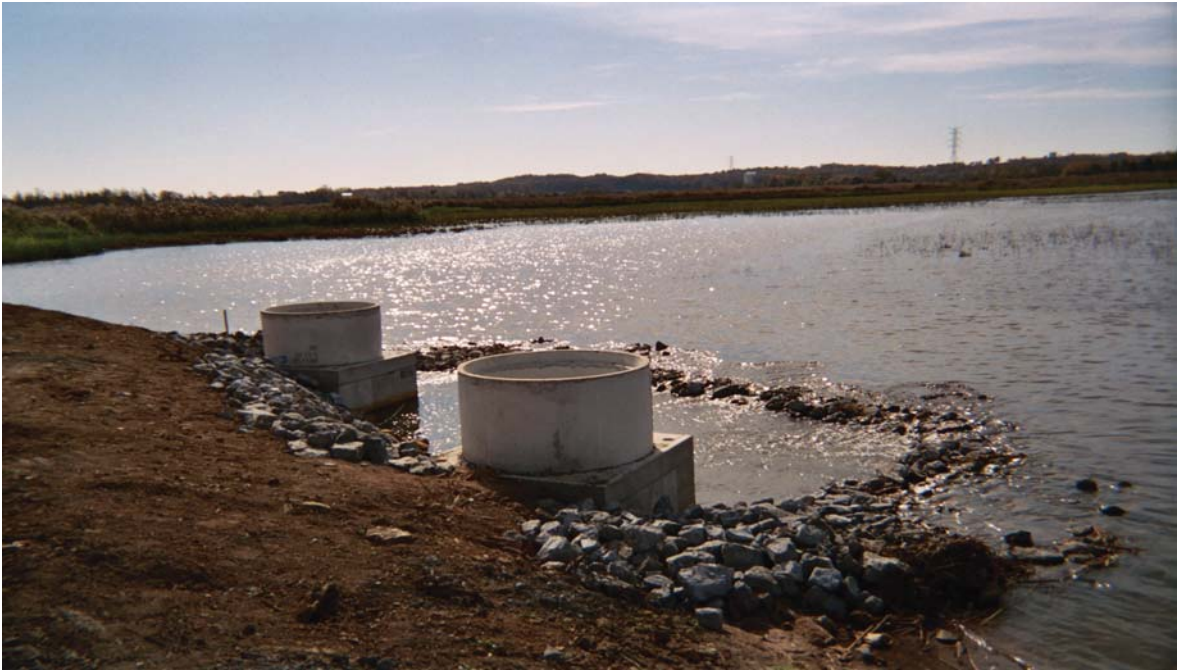
Picture 7: New drainage structures from Pond E to Pond D
