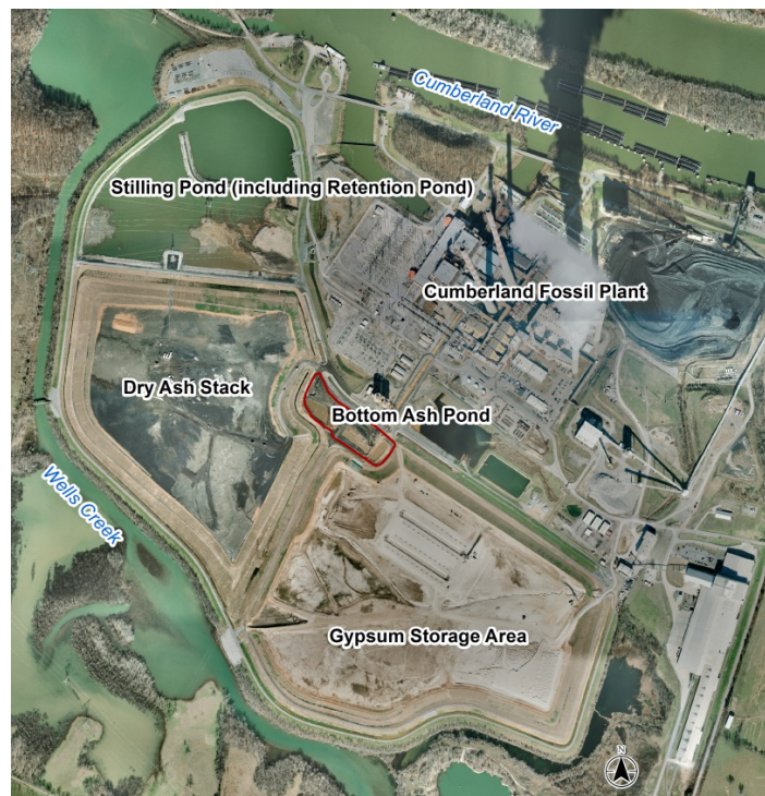
Figure 1 Bottom Ash Pond Approximate Boundary
