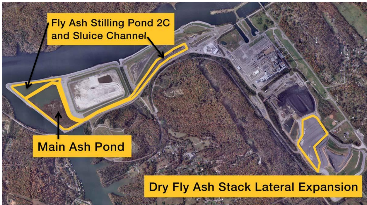
Figure 1: Ash Pond Complex
