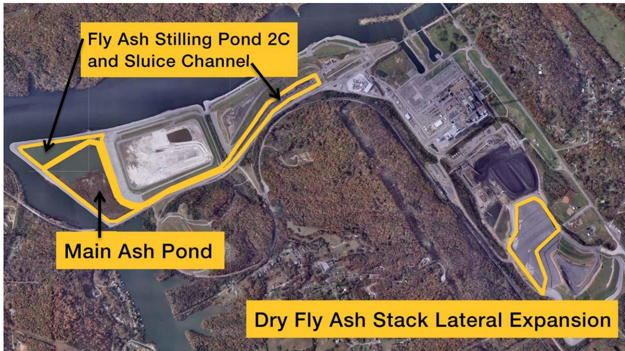
Figure 1: Ash Pond Complex
