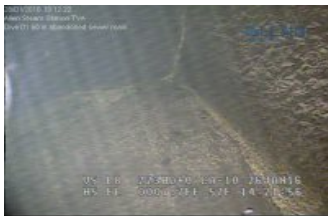
190 ft from manway 17 note derbis at side wall of pipe_C1.jpg
