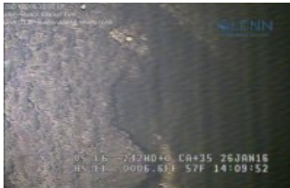
125 ft from manway 17 buildup on pipe wall left springline_C1.jpg
