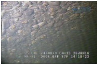
155 ft from manway 17 exposed aggregate at 10 O'clock position_C1.jpg
