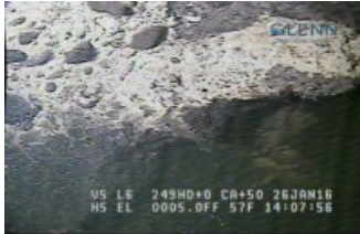
120-feet from manway 17 buildup at crown of pipe_C1.jpg
