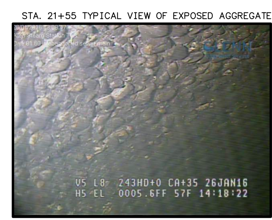
STA. 21+55 TYPICAL VIEW OF EXPOSED AGGREGATE
