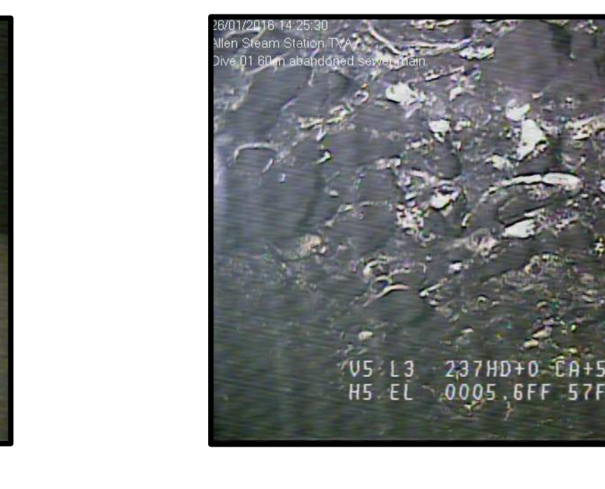
STA. 33+90 TYPICAL VIEW OF EXPOSED AGGREGATE
