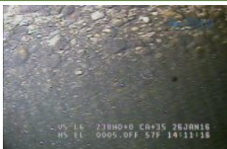
150 ft example of exposed aggregate at crown of pipe_C1.jpg
