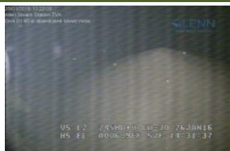
295 ft from manway 17. Sand deposit at invert of pipe. below joint. C1.jpg
