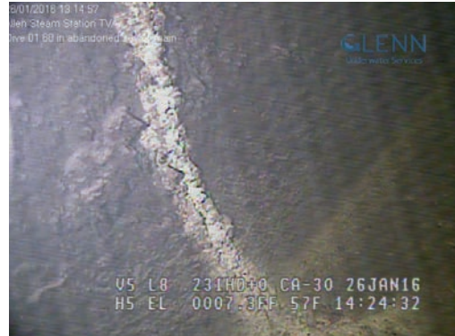
Figure 4 – 213" downstream from manhole No. 17. View of joint with calcite material.
