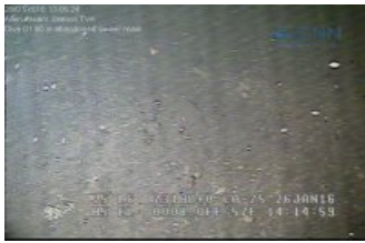
145 ft from manway 17 view of silt at invert of pipe_C1.jpg
