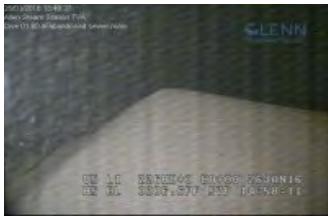
810 ft from manway 17 large amount of debris at invert of pipe C1.jpg
