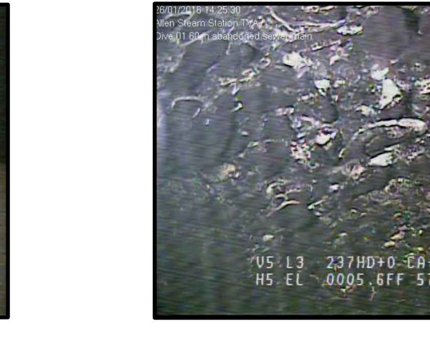
STA. 33+90 TYPICAL VIEW OF EXPOSED AGGREGATE
