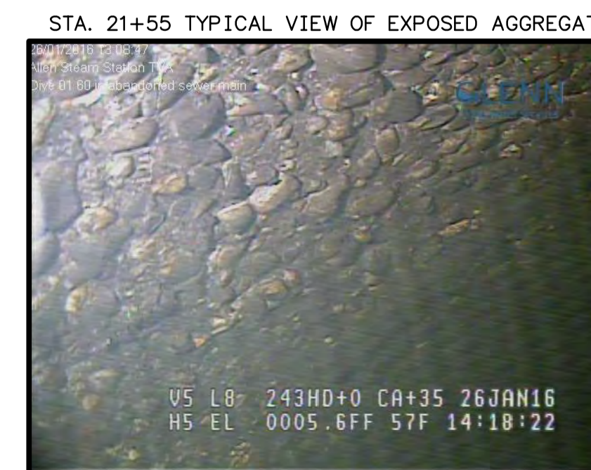
STA. 21+55 TYPICAL VIEW OF EXPOSED AGGREGATE
