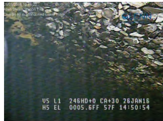
Figure 3 – 800' downstream from manhole No. 17. Example of exposed aggregate with loose cement paste.
